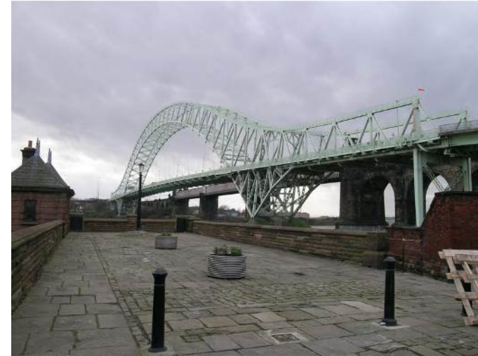
Existing Silver Jubilee Bridge
